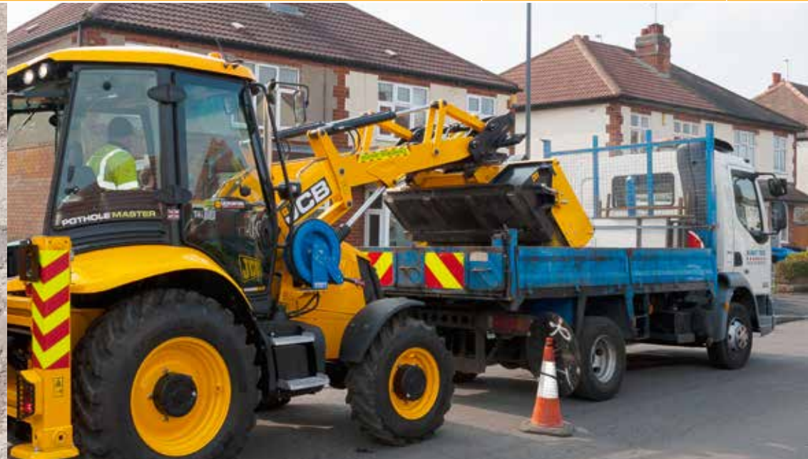
5. TIDY UP | Empty all debris into truck and move to next job.
