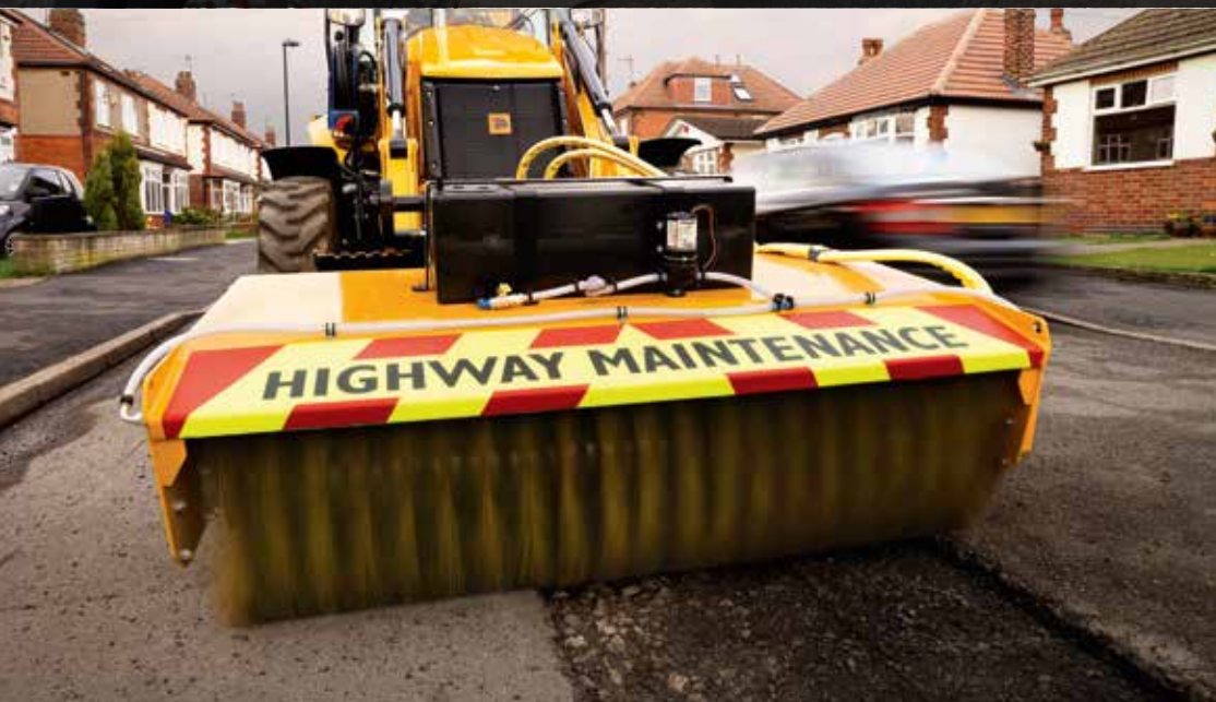
4. SWEEP OUT | The sweeper collector picks up all debris, dirt and water.
