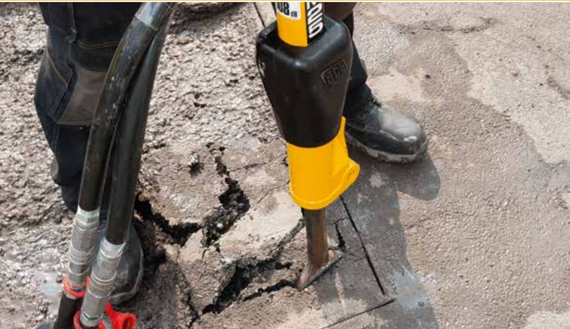
3. BREAKING | Attach a handheld breaker to finish off and save time.
